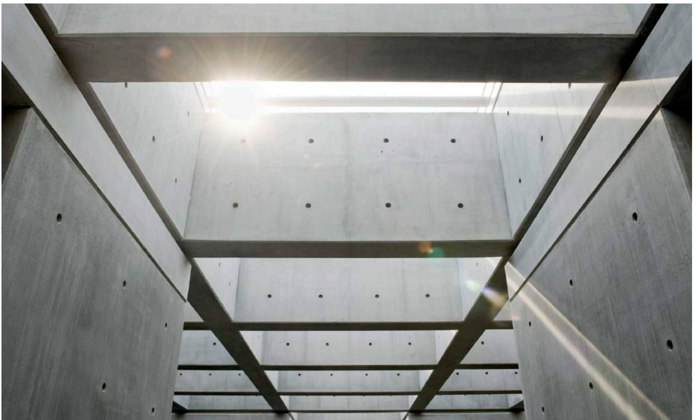
Atrium roof coffer
