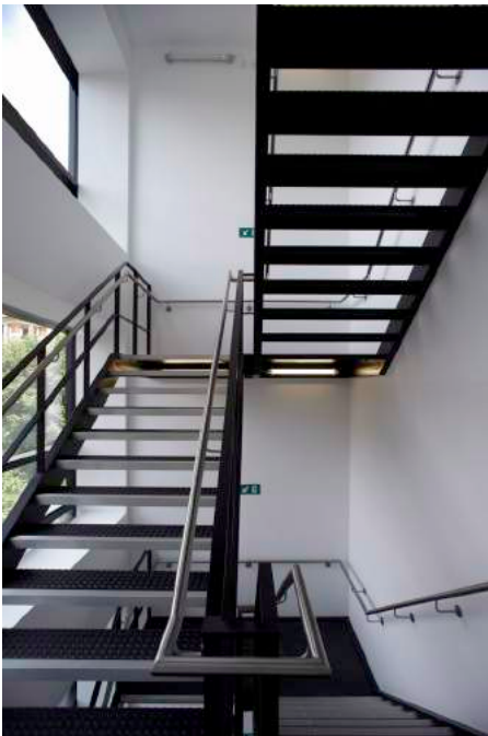
North circulation stair
