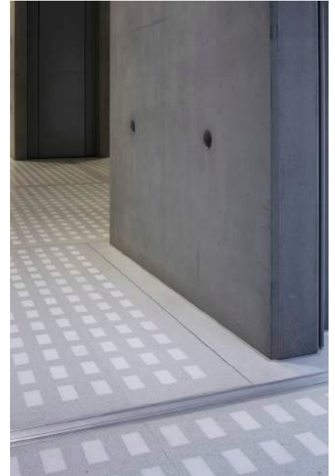
Movement joint in terrazzo floor
