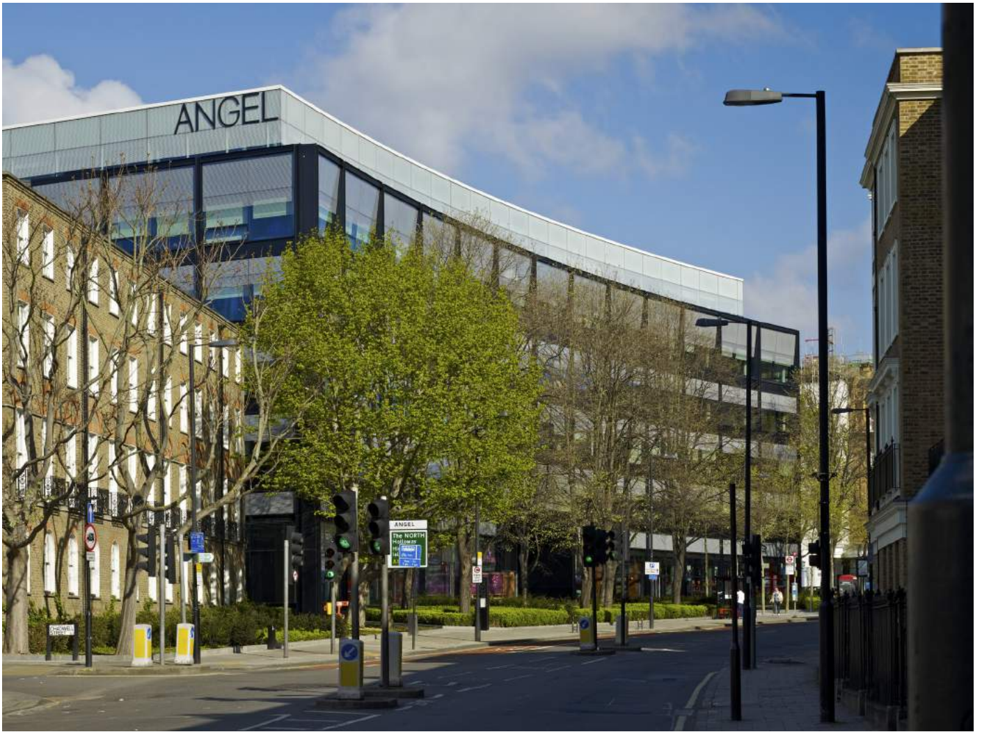
Angel Building from St. John Street
