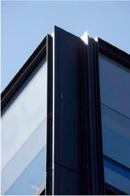
Cladding corner junction
