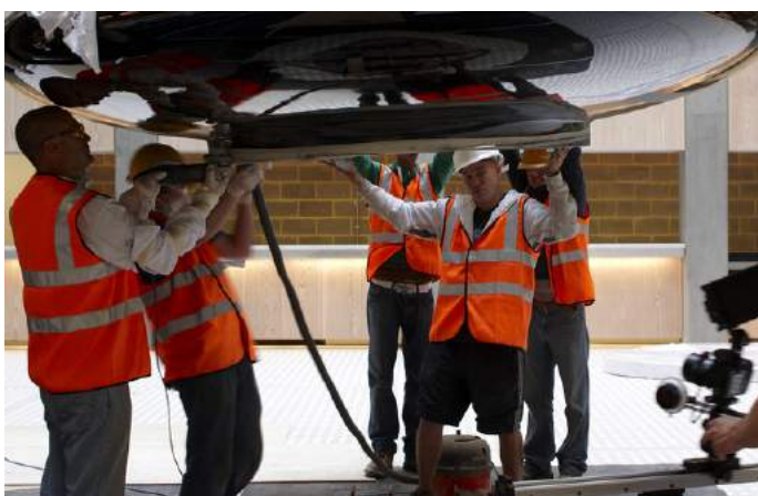
Installation of base element in progress
