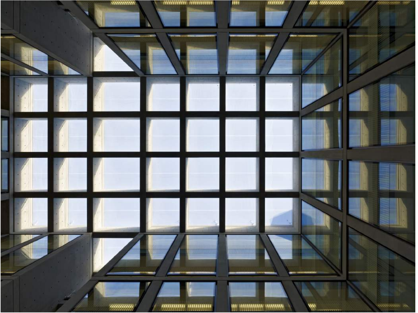
Main atrium roof coffer viewed from ground floor
