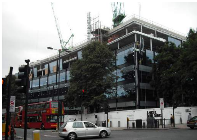
North & east elevations in progress, August 2009
