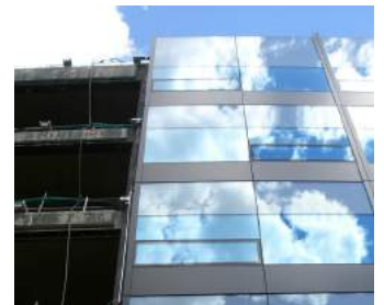
West elevation in progress
