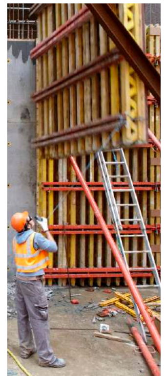
Contractor placing formwork
