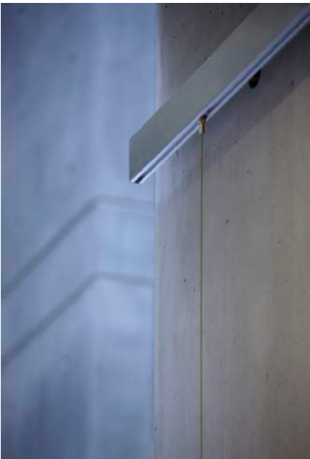
Bespoke picture rail fixed into tie holes
