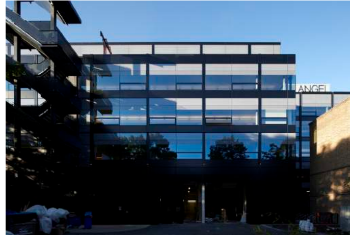
The solar coating in the glass gives it its blue hue
