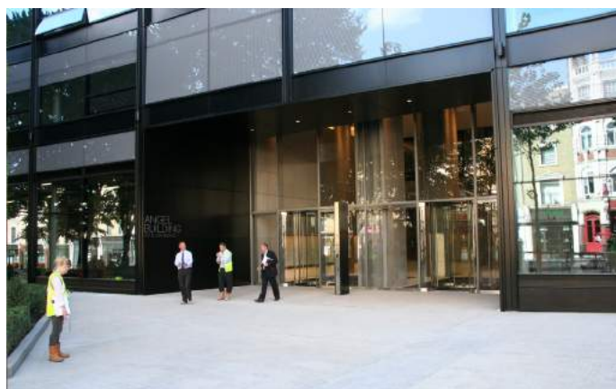
Entrance portal at practical completion, August 2010
