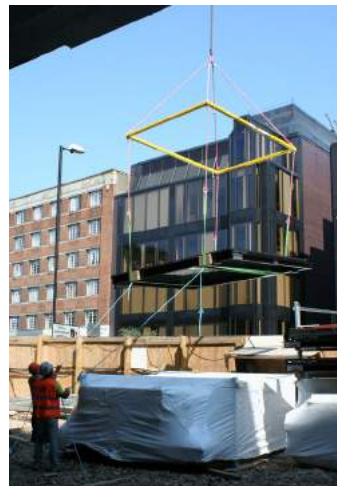
Lifting of panel for installation
