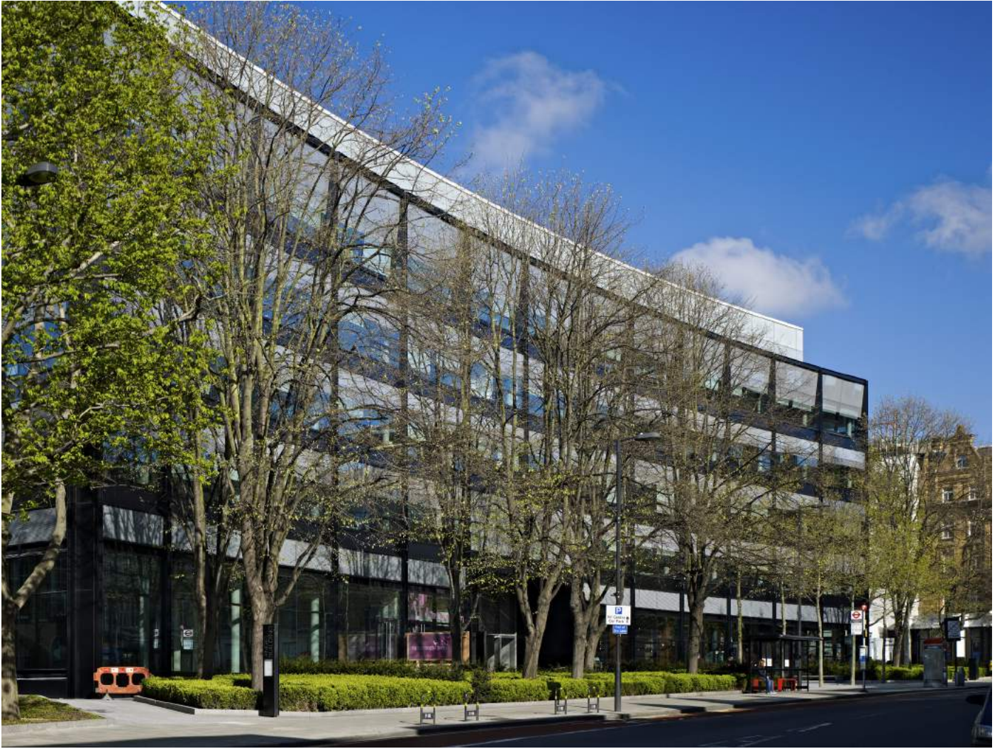
Angel Building from St. John Street
