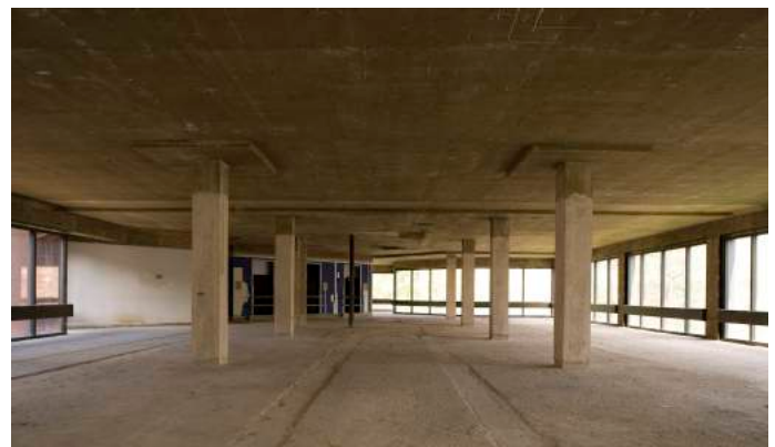
Views of structure post strip-out
