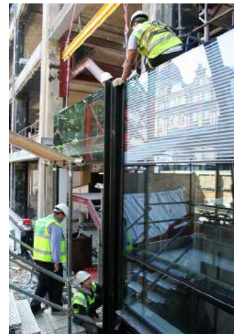
Installation of ground floor panels
