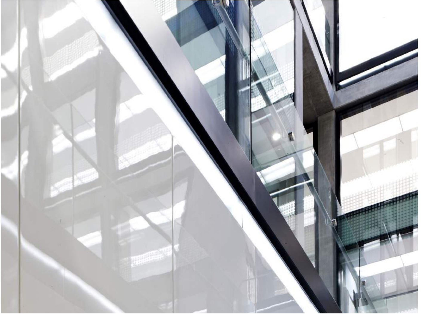
Detail of glazing
