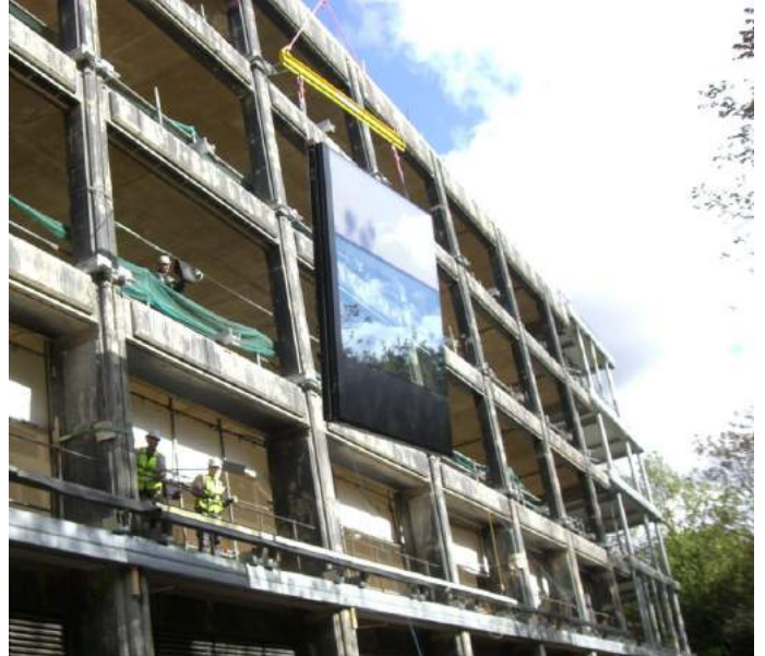
May 2009. Installation of first panel, west elevation
