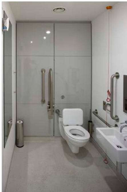
Wheelchair accessible WC
