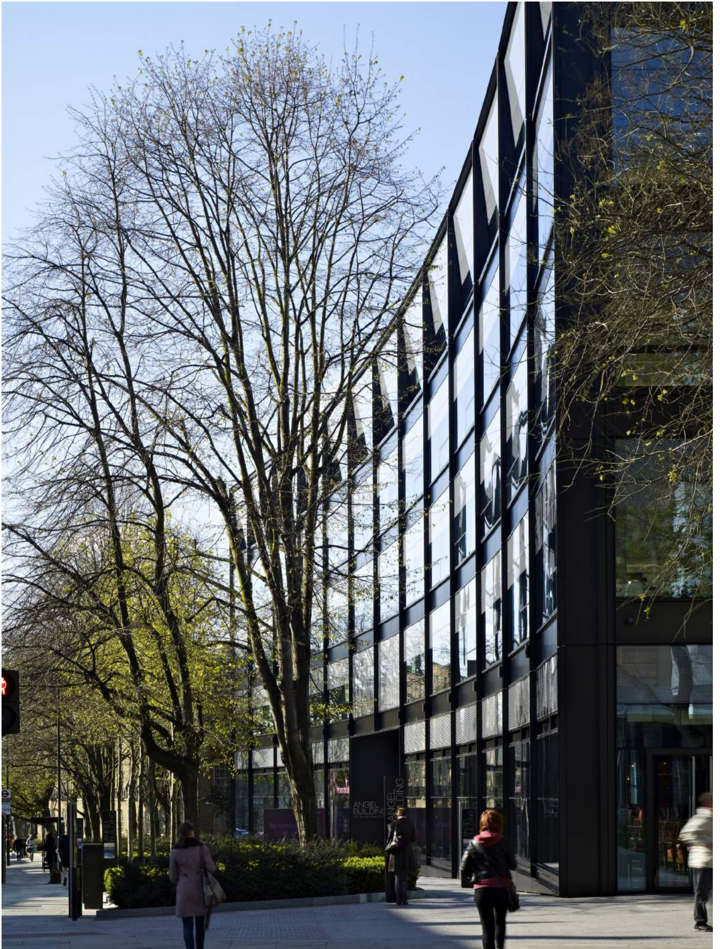
View from the corner of Pentonville Road
