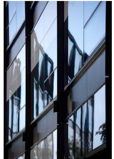
Integrated external lighting
