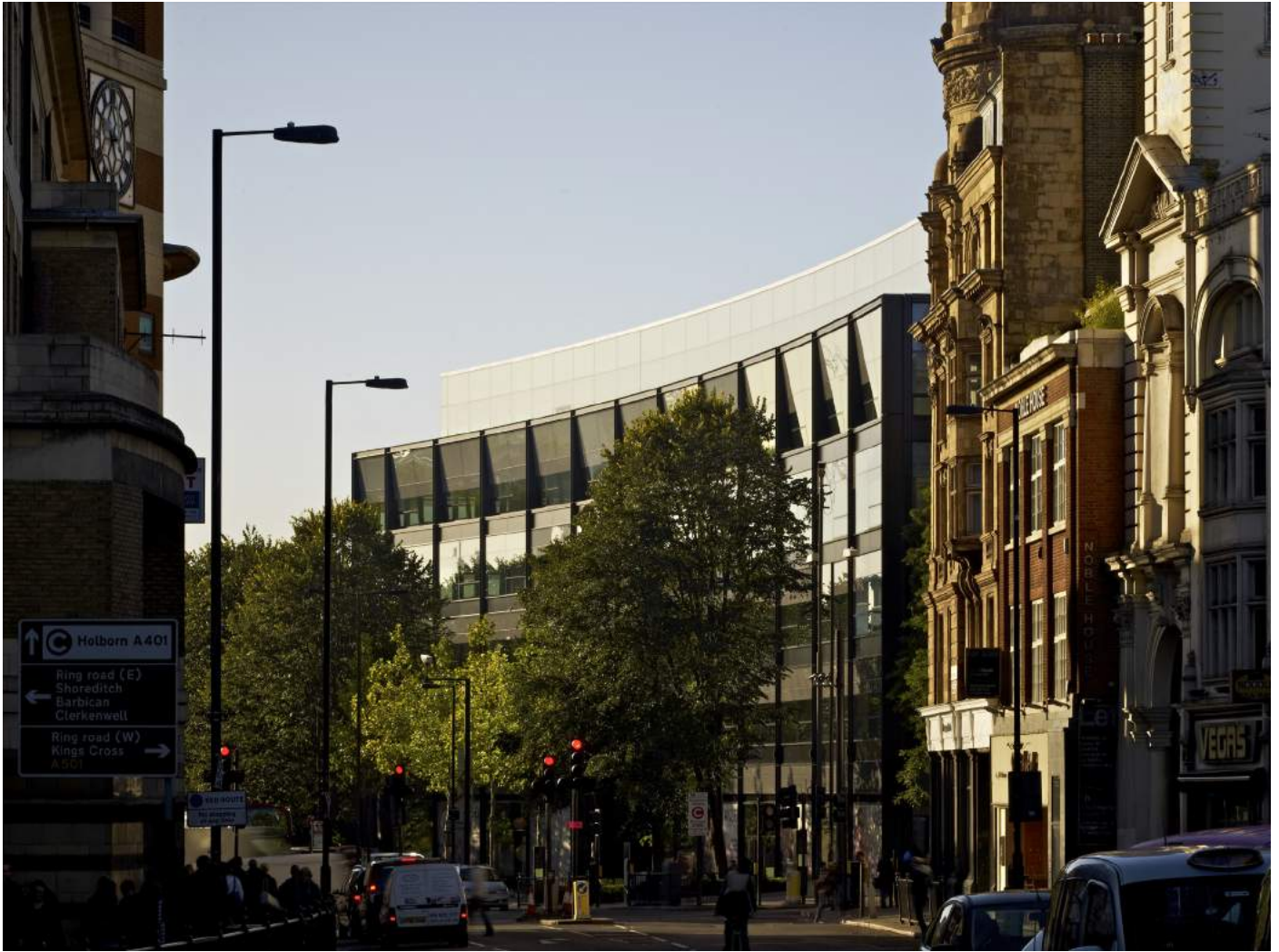
View of completed façade from Angel Underground station
