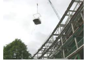
Lifting of crates to store location
