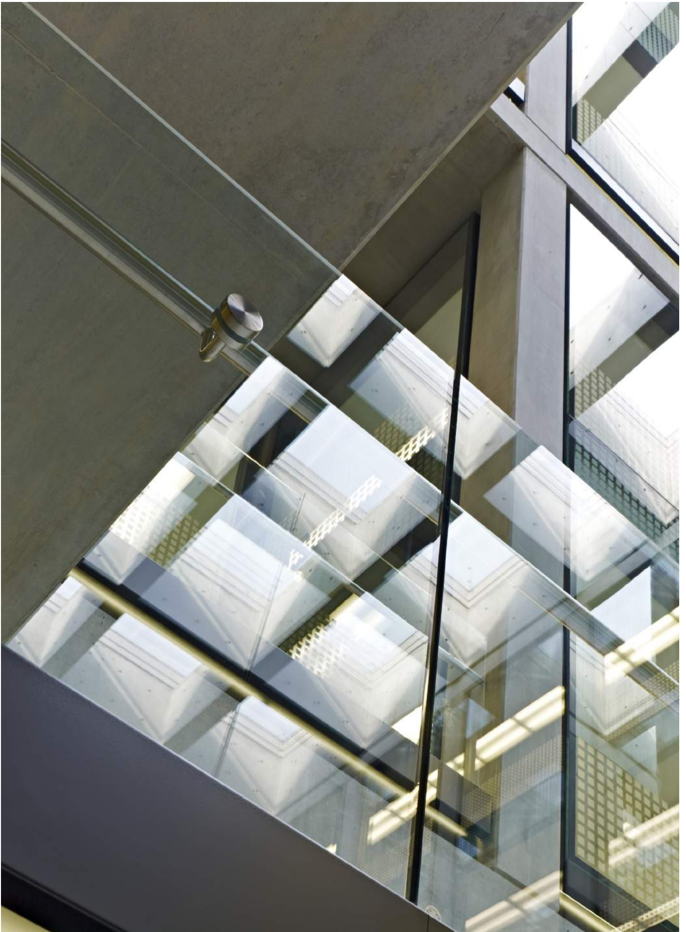
Detail of glazing
