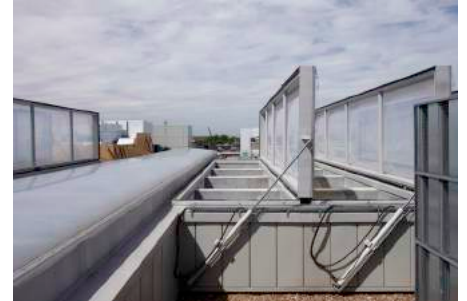
ETFE roof open
