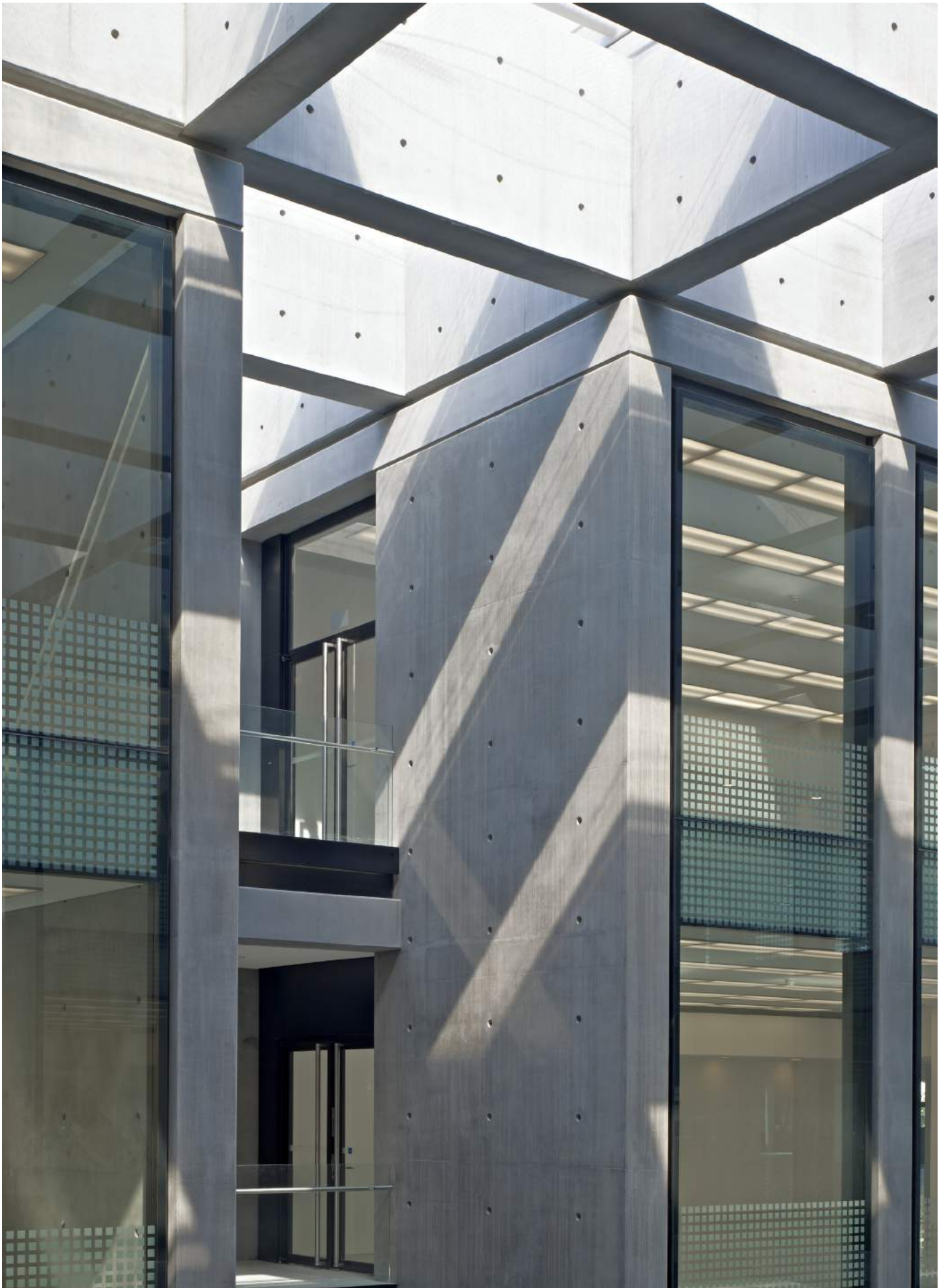
Atrium cladding alongside the concrete fin walls
