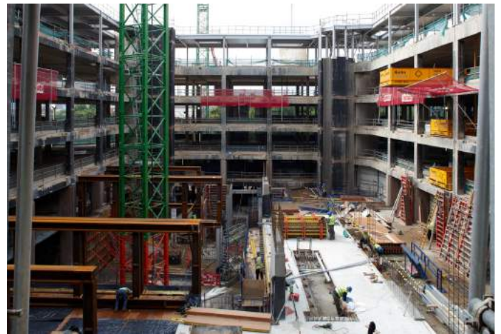
The atrium during construction, June 2009
