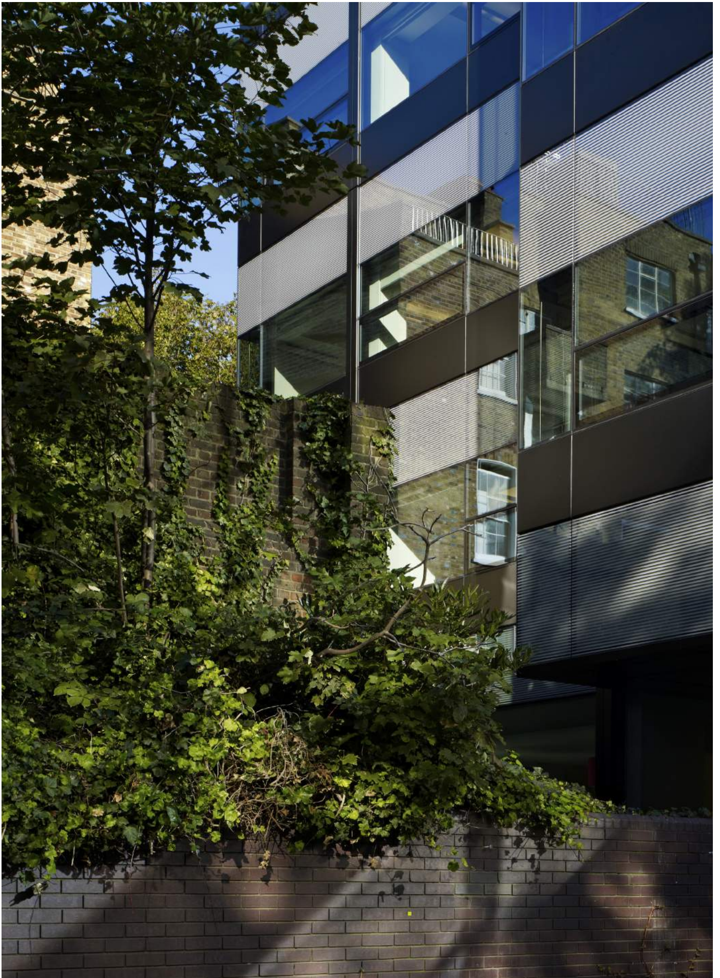
Detailing of west façade
